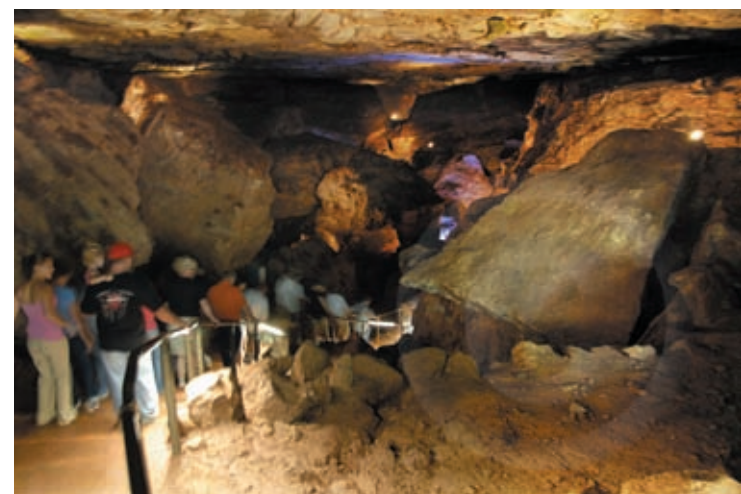
A project providing lighted handrails and other lighting has just been completed in the caverns. - Indexfoto
