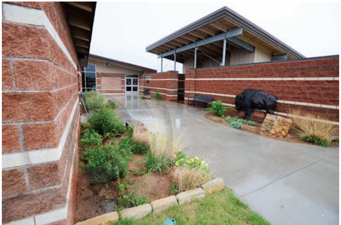
The new park headquarters and interpretive center at Caprock Canyons State Park was built in October, 2007. It is located just three miles north of Quitaque in Briscoe County.
