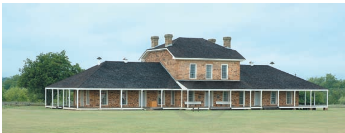
The completely restored hospital and morgue, largest of the buildings dating from the 1860's inside Fort Richardson State Park.
