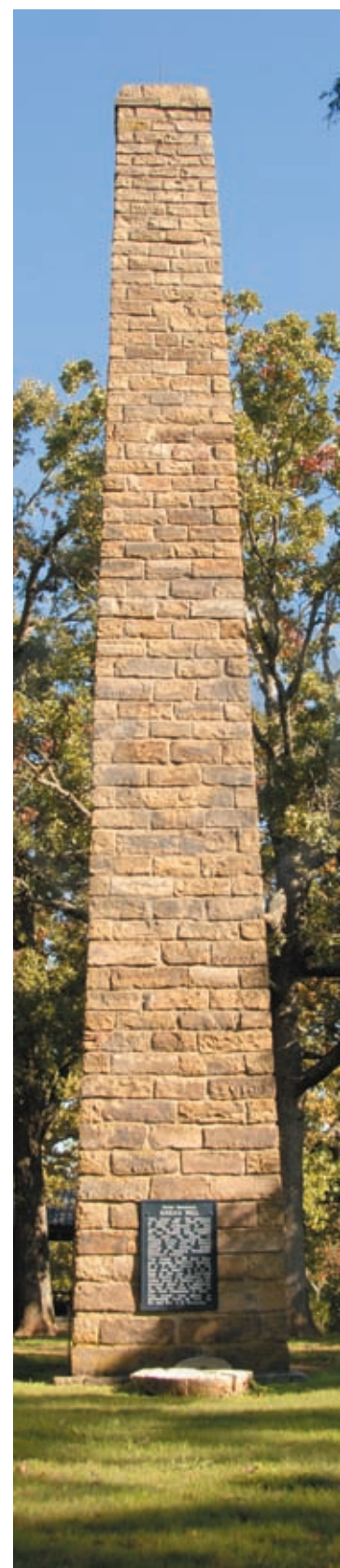
THIS 70,000-TON BATTLE MONUMENT was the chimney from a steam-powered mill at nearby Rhea, Arkansas, and was dedicated to all who fought at Prairie Grove. - Indexfoto
